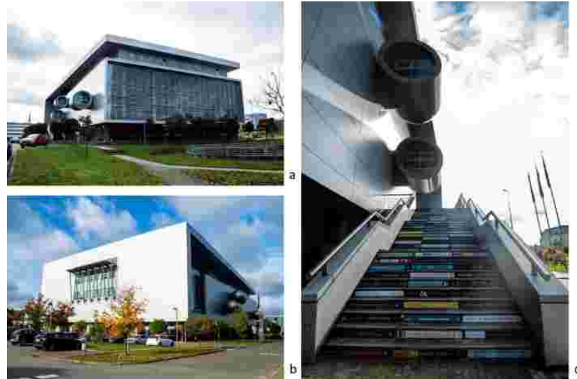
Figure 1.6. the exterior of the UG main library consisting of the pictures of northeast façade (a), southeast façade (b), and the stairs on the northwest façade (c) (Pictures by Mosleh Ahmadi).
